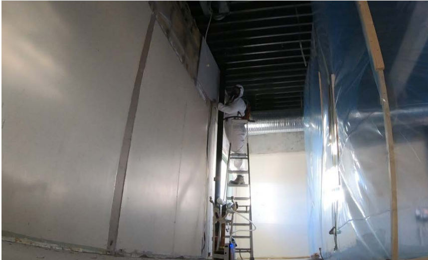
Figure 3.1: Removal of indoor asbestolux wall plates
