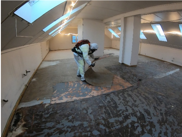
Figur 3.2: Removal of asbestos containing floor.
