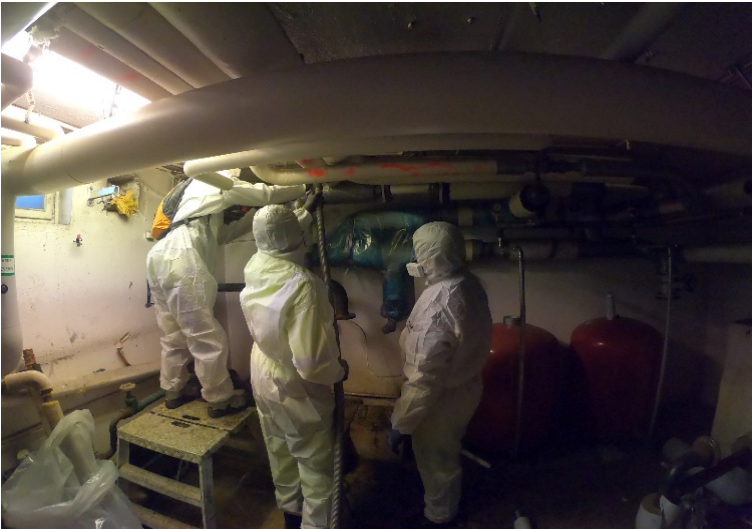
Figure 3.5: Removal of a pipe section with asbestos insulation.
